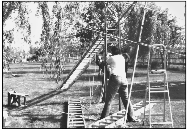
Fig 6—Walking the ladder up to its vertical position. Keith, VE2AQU, supports the mast with a second ladder while Chris, VE2FRJ, checks the ropes. (Photo by Keith Baker, VE2XL.)
