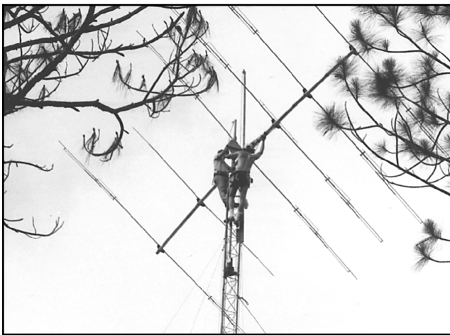
Fig 42—The U bolts securing the short pipe to the mast plate are loosened and the boom is turned to a horizontal position. This puts the elements in a vertical plane. Then the pipe U bolts are tightened and pinning bolts secured. The boom U bolts are then loosened and the boom turned axially 90°.
