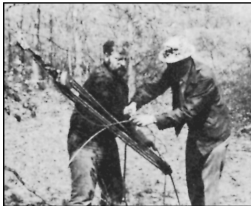
Fig 23 —Proper tension can be placed on the guy wires with the aid of a block-and-tackle system. (Photo by K1WA)
