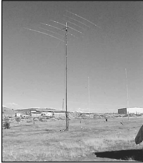
Fig 18—Installation of surplus AB-577 tower with tribander at 45 feet at K7NV. (Photo by Kurt Andress, K7NV.)
