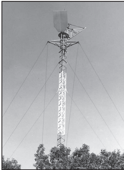
Fig 81—Commercial periscope antennas, such as this one, are often used for point-to-point communication.
